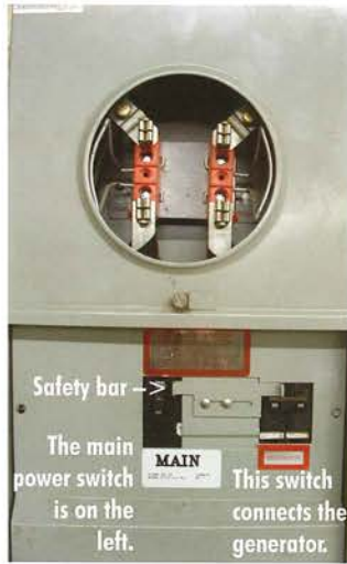
In this photo, the safety bar, which is locking out the generator switch, prevents backfeeding to the power lines.
